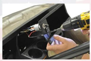
9. Using a 7/16 drill bit, drill out the hole for the Push/Pull switch. Drill gently.
